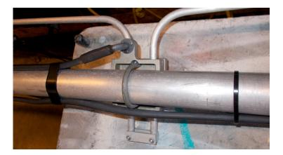
A MIG unit for aluminum was located for the Author to use, which had only 5 minutes of experience about 30 years ago. Therefore, it was a little ugly but should be strong enough to hold up with the high winds at the site. Shown here is the hole drilled for the bolt, washer and nut to be installed.
